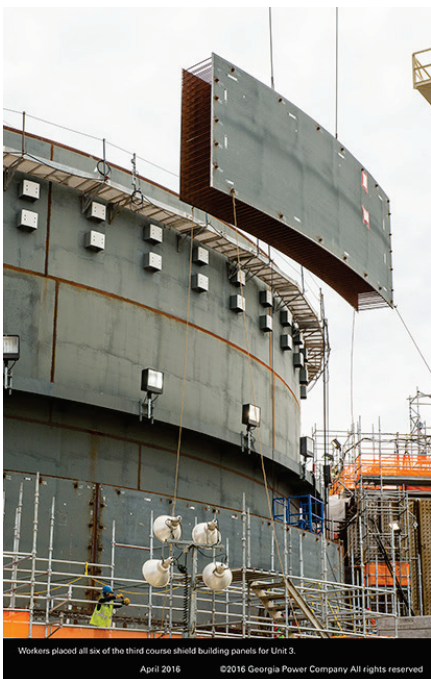
Vogtle Unit 3 – AP1000, United States, April 2016 (Georgia Power Company, all rights reserved).
