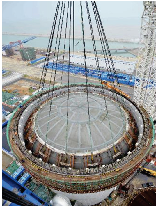
Haiyang Unit 2 – AP1000, China, August 2015, CVTH Installation (provided by NNSA).
