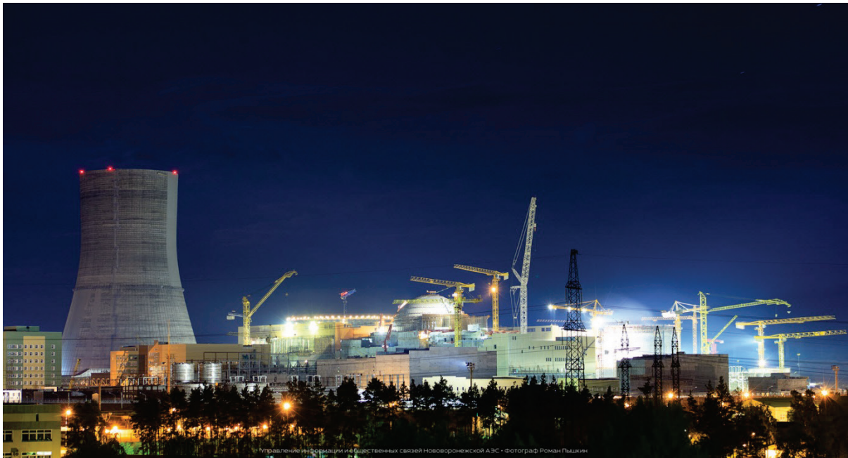
Novovoronezh NPP-2 – Overview of the construction site, VVER, Russia, 2016 (provided by Rostekhnadzor).
