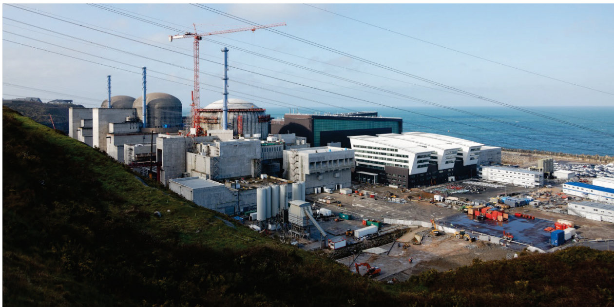
Flamanville 3 – Construction site aerial view, EPR, France, 24 March 2016 (© EDF All rights reserved. Aménagement Flamanville 3, Communication).
