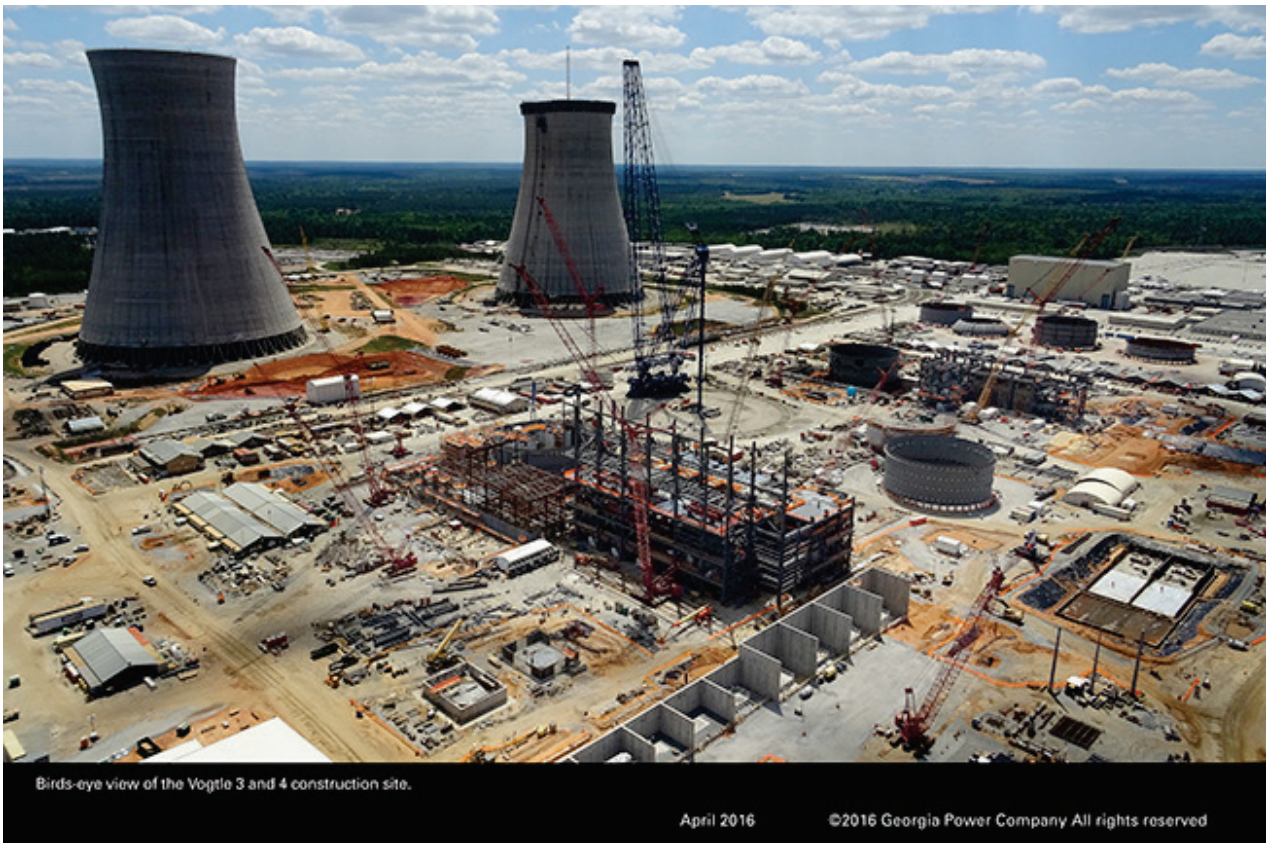
Vogtle Unit 3 and 4 – Aerial view, AP1000, United States, April 2016 (Georgia Power Company, all rights reserved).
