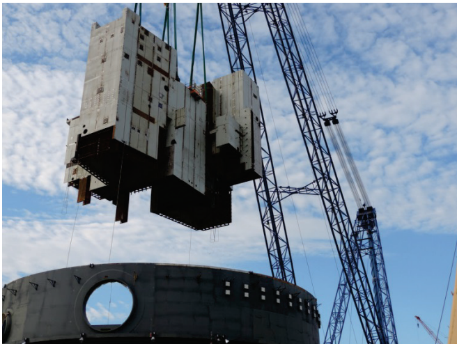
V.C. Summer Unit 2 – Installation CA01 in containment, AP1000, United States, 23 July 2015 (SCE&G, all rights reserved).
