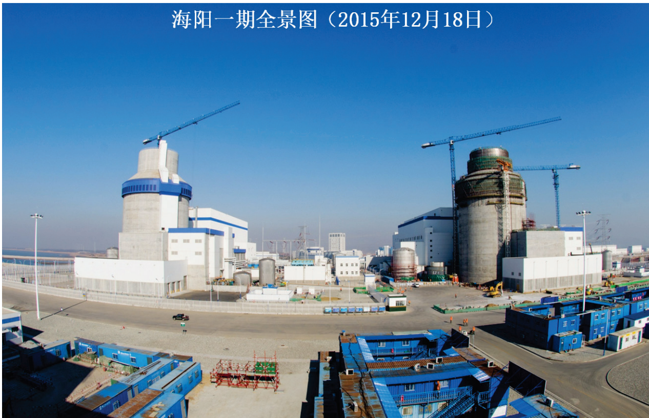
Haiyang Units 1 and 2 – Construction site, AP1000, China, 18 December 2015 (provided by NNSA).
