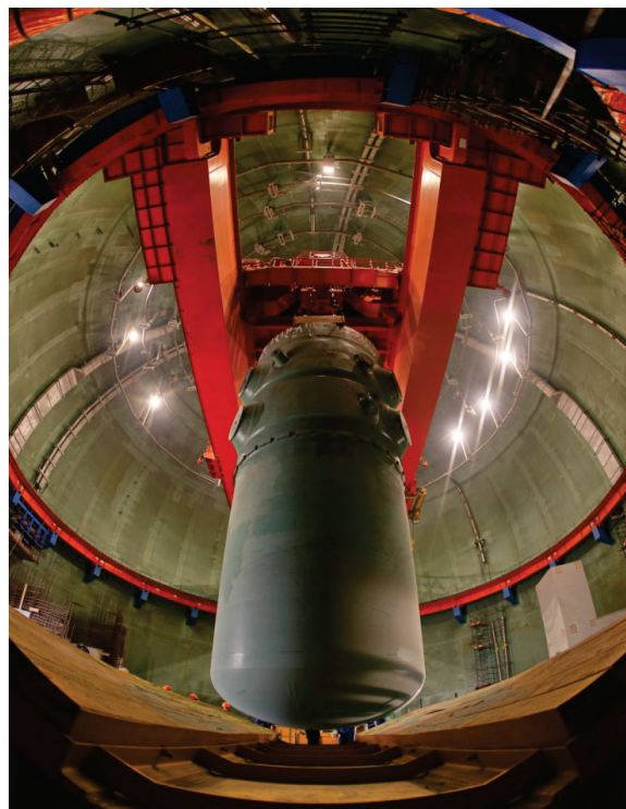
Tianwan NPP Unit 4 – RPV lifted in position 17 March 2016, VVER, China (provided by NNSA).
