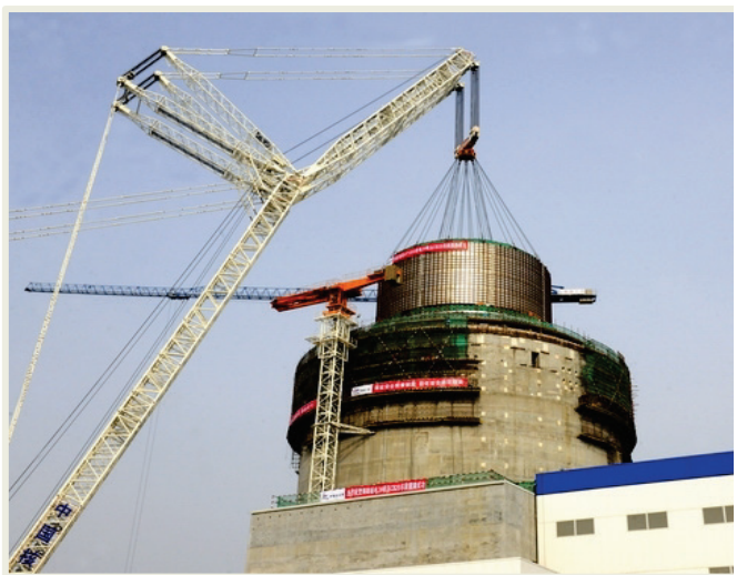
Sanmen Unit 2 – AP1000, China, December 2015, CB20 Hoisted in Place (provided by NNSA).
