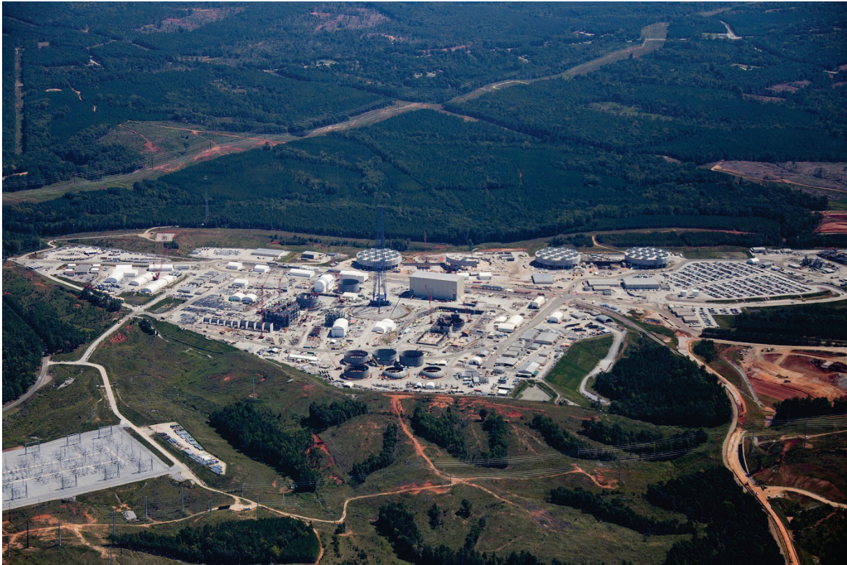
V.C. Summer – Units 2 and 3 AP1000 Construction Site Aerial View – United States, September 2015 (SCE&G, all rights reserved).
