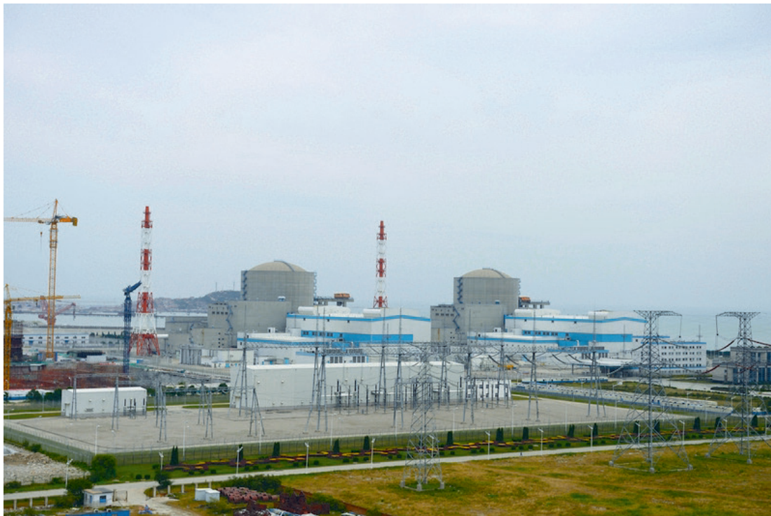
Tianwan NPP Unit 3 and 4 – Construction Site VVER, China, 2016 (provided by Rostech nadzor).
