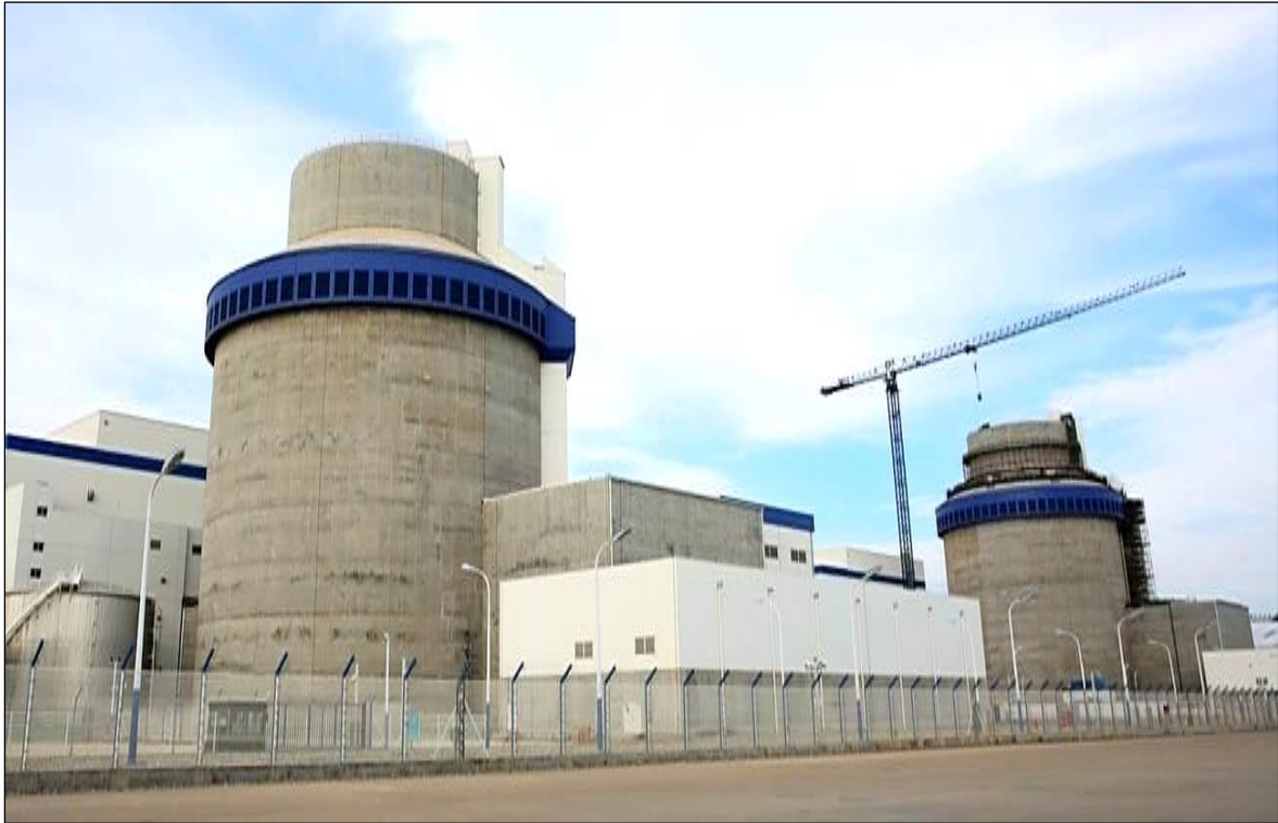
Haiyang Unit 2 – AP1000, China, September 2017, CVTH Installation (Provided by NNSA).
