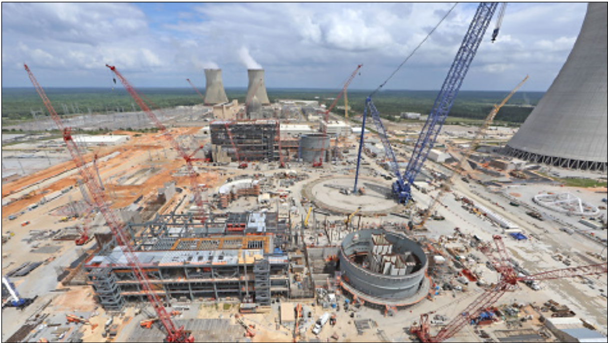
Vogtle Unit 3 and 4 – Aerial view, AP1000, United States, April 2017 (Georgia Power Company, all rights reserved).
