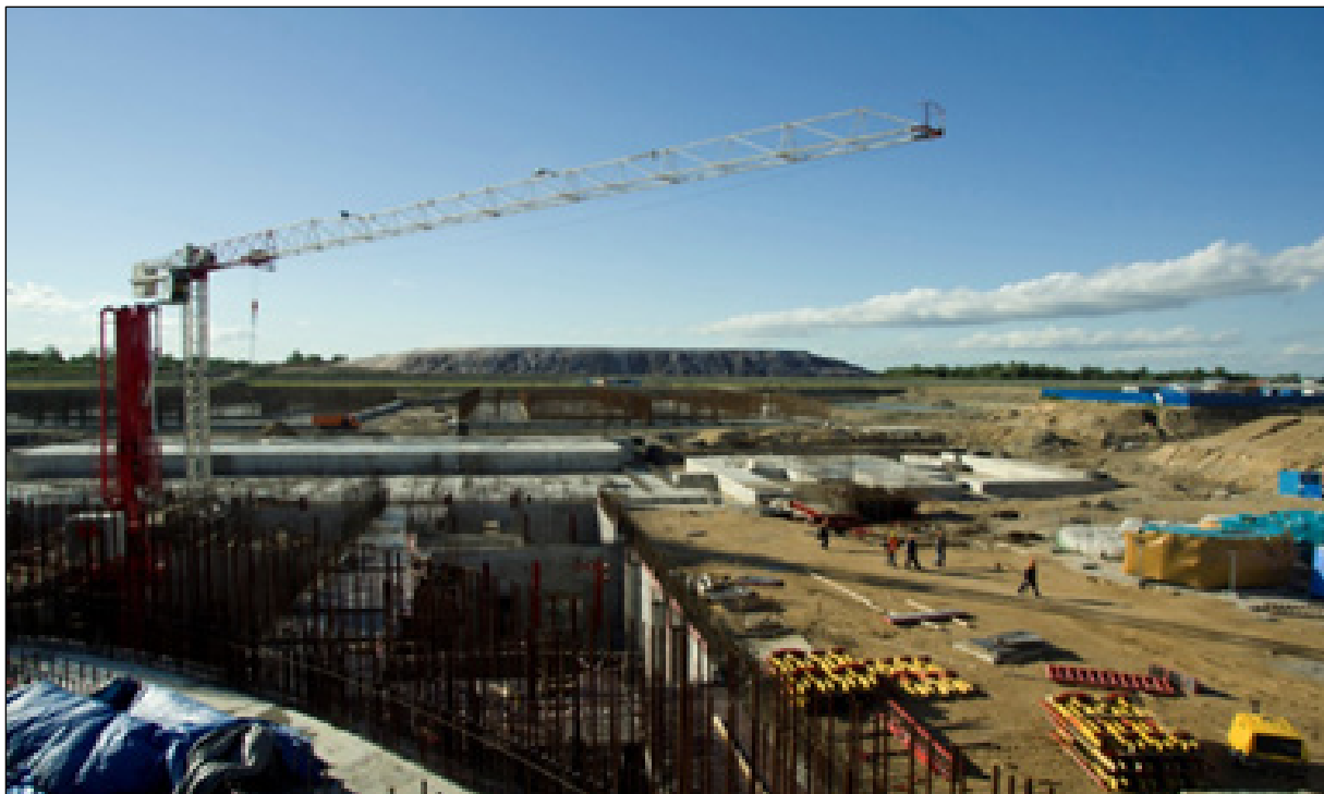
Baltic NPP-2 Unit 1 – Overview of construction site, VVER, Russia, 2016 (Provided by Rostekhnadzor).
