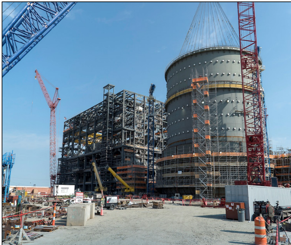
V.C. Summer Unit 2 – Placed final Unit 2 containment vessel ring, AP1000, United States, 9 June 2017. (SCE&G, all rights reserved).
