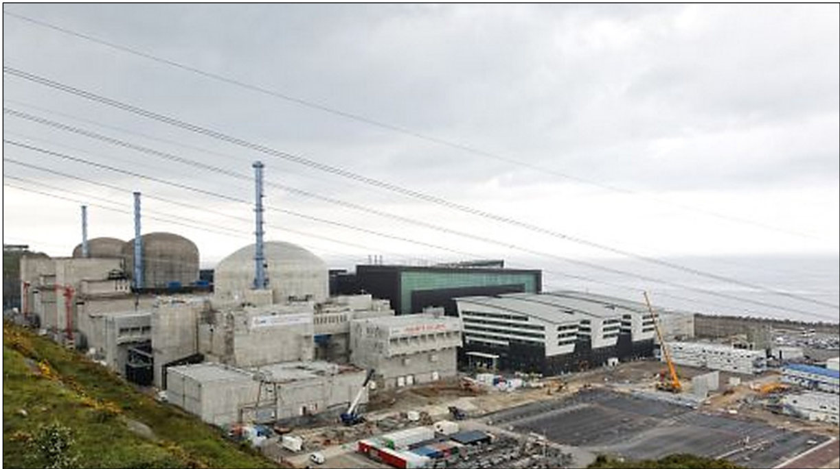
Flamanville 3 – Construction site aerial view, EPR, France, 31 May 2017 (© EDF All rights reserved. Aménagement Flamanville 3, Communication).
