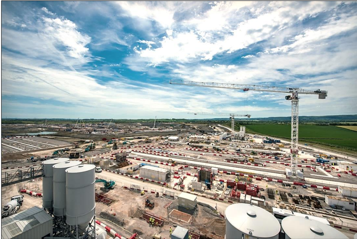
Hinkley Point C – View from the Batching Plants, showing the Bylor fabrication area, tower cranes, and Kier BAM JV spray concrete batch plant, EPR, UK. May 2017 (Provided by EDF).
