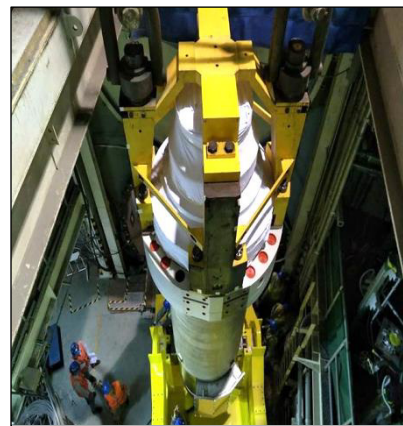
Sanmen Unit 2 – AP1000, China, RCP installation (Provided by NNSA).
