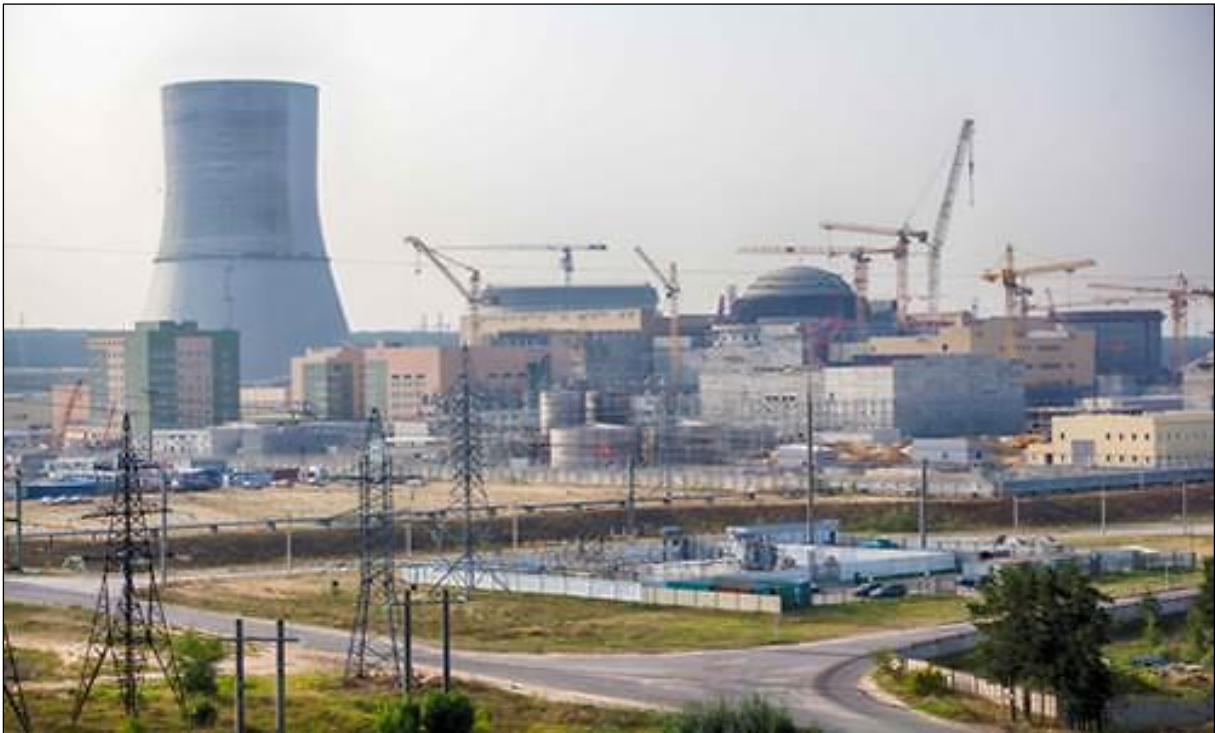
Novovoronezh NPP-2 Unit 1 – Overview, VVER, Russia, 2016 (Provided by Rostekhnadzor).
