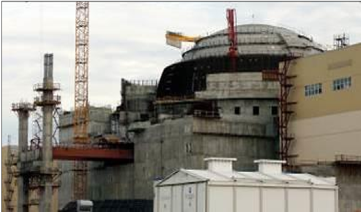
Novovoronezh NPP-2 Unit 2 – Overview of construction site, VVER, Russia, 2016 (Provided by Rostekhnadzor).
