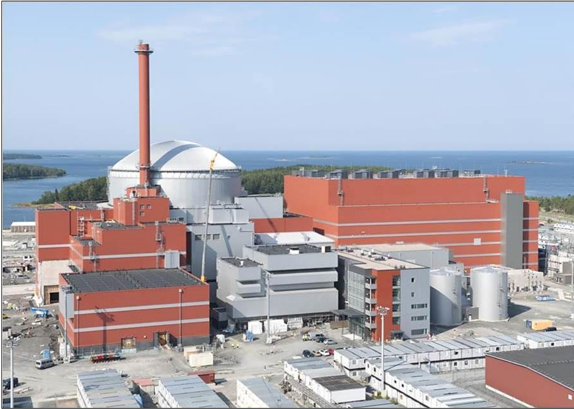
Olkiluoto 3 – EPR, Finland, May 2016 (Provided by STUK).
