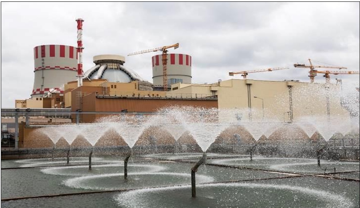
Novovoronezh NPP-2 Unit 1 – Overview, VVER, Russia, 2016 (Provided by Rostekhnadzor).
