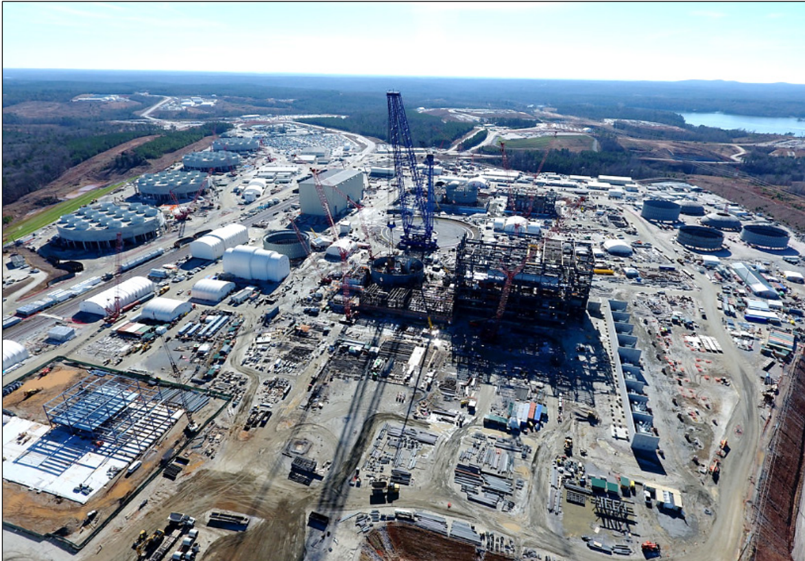
V.C. Summer – Units 2 and 3 AP1000 Construction Site Aerial View – United States, January 2017. (SCE&G, all rights reserved).
