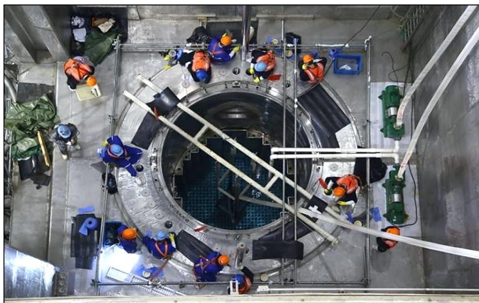
Sanmen Unit 1 – AP1000 China, April 2016 Installation of HFT. (Provided by NNSA).
