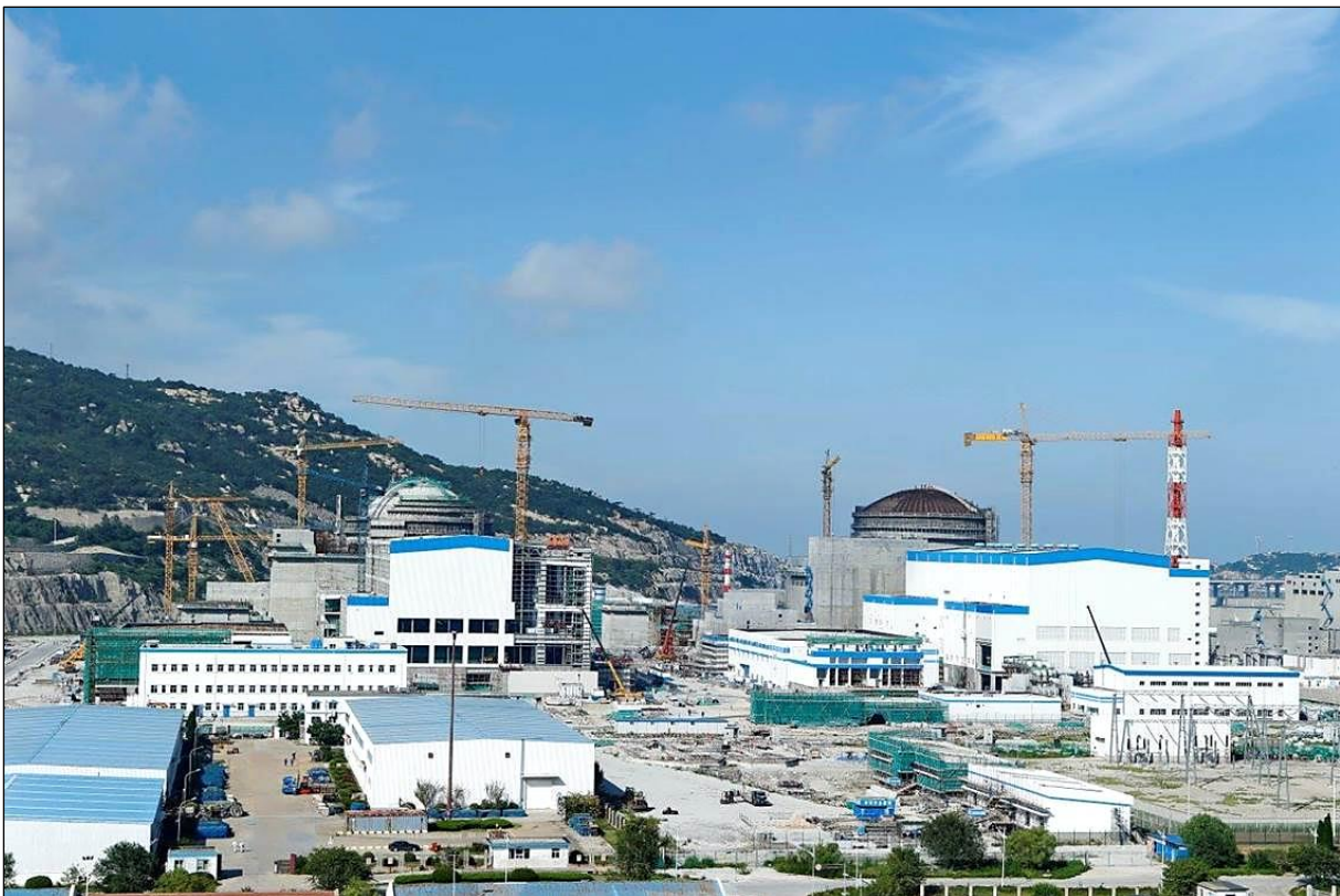
Tianwan NPP Unit 3 and 4 – Construction Site VVER, China, 2016 (Provided by NNSA).
