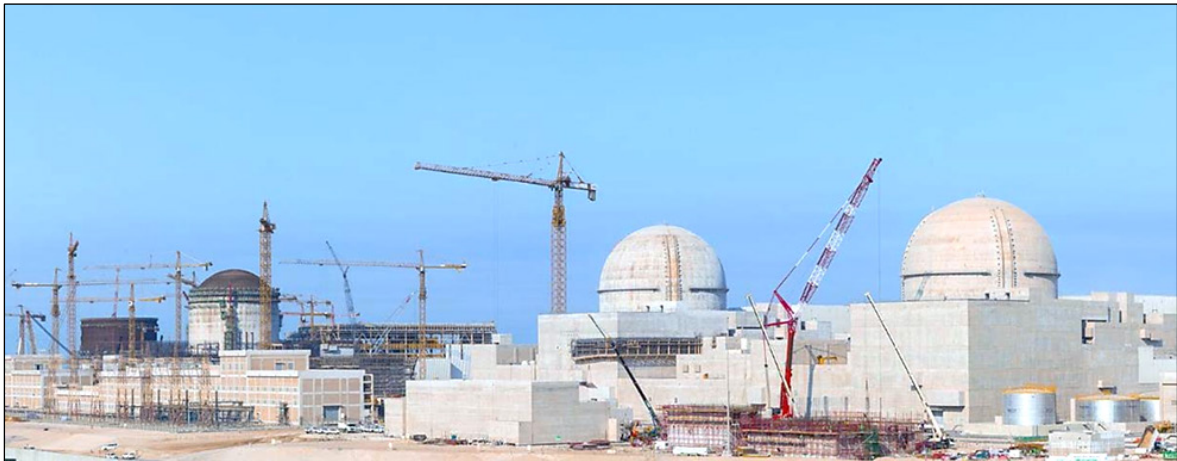
Barakah Units 1,2,3, 4 – Overview, APR1400, United Arab Emirates, February 2017 (Property of ENEC).
