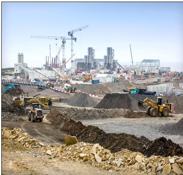
Hinkley Point C – North West Area of Construction Site, EPR, UK, May 2017( Provided by EDF).
