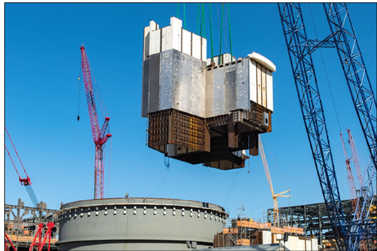
Vogtle Unit 4 – AP1000, United States, August 2016 CA20 module placed (Georgia Power Company, all rights reserved).
