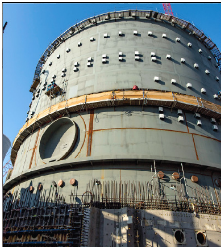
Vogtle Unit 3 – AP1000, United States, December 2016 Middle Ring placed in nuclear island (Georgia Power Company, all rights reserved).
