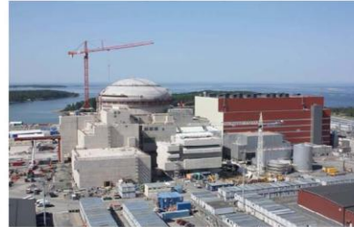
EPR™ reactor construction site, Olkiluoto (Finland), 2011, July
