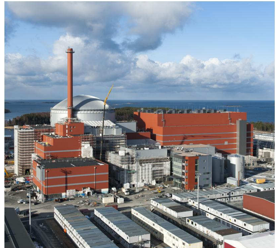
Olkiluoto 3 in March 2014. Picture: TVO
