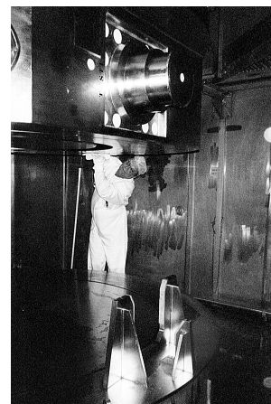
F: Decontamination of rear part
