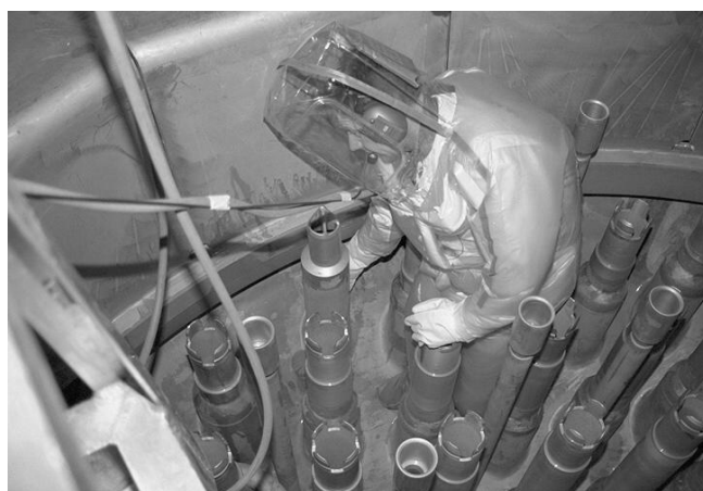
Picture 2. Picture of the bottom nozzles of the reactor pressure vessel
