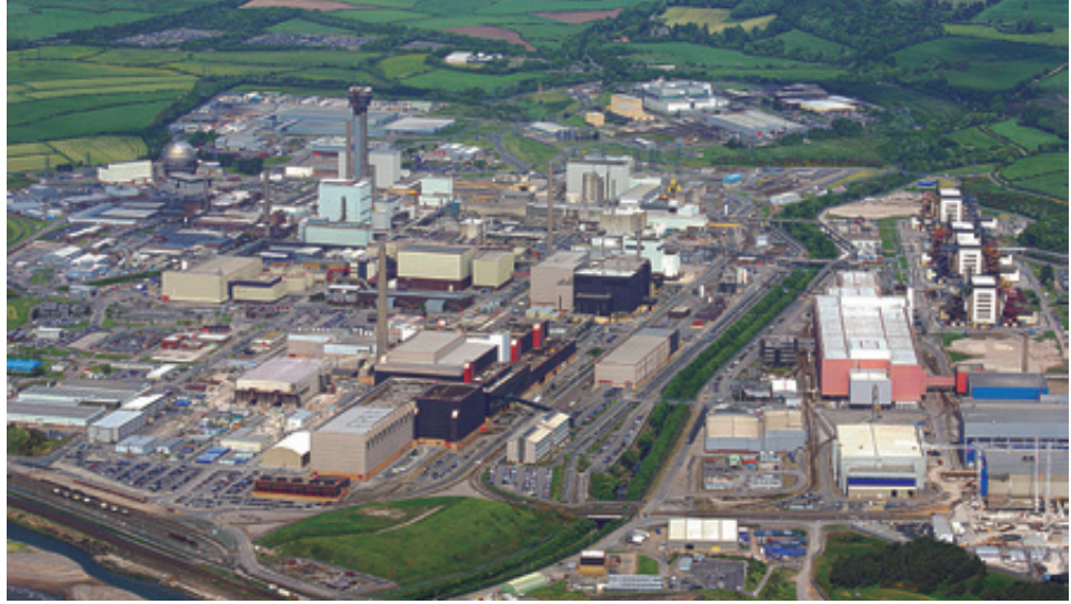
Aerial view of the Sellafield site, Sellafield, United Kingdom.
