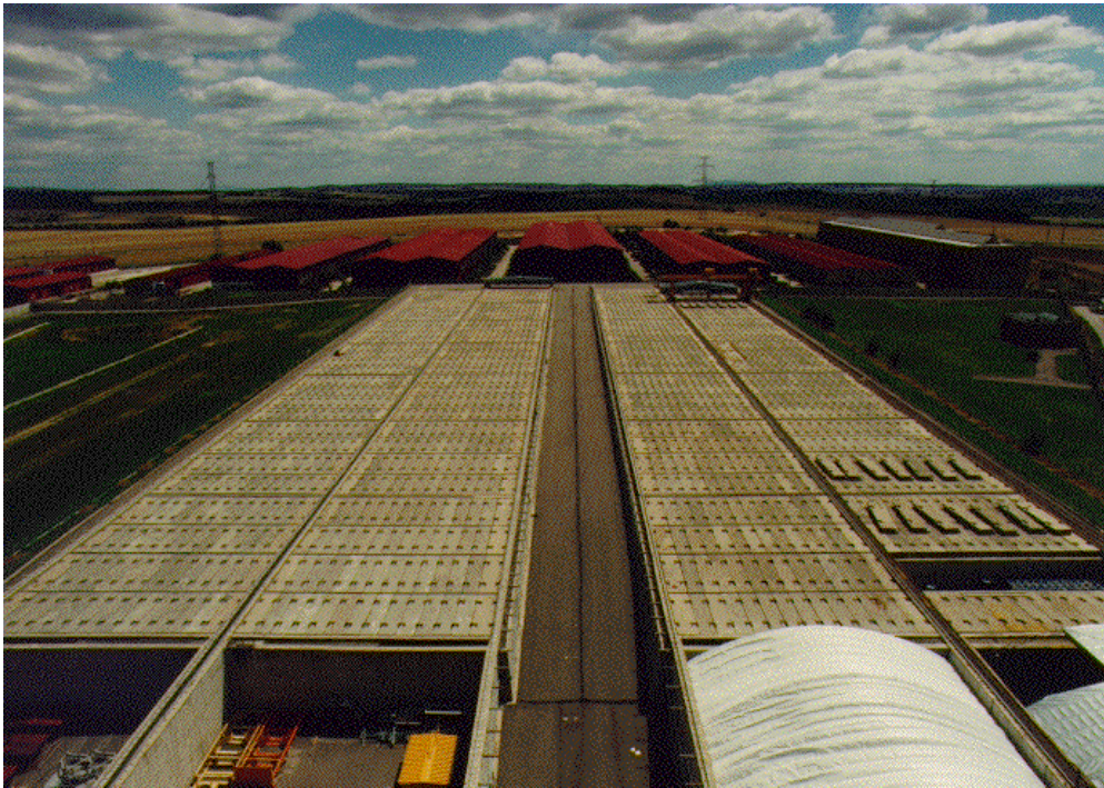
Figure A2.2 Dukovany LLW and ILW Repository
