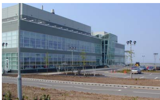
Figure 8.1: External view of Central Laboratory, Sellafield
