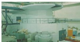
DD&R tech. for research reactor and uranium conversion plant
