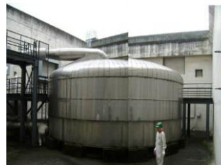
Existing FCV reinforcement
