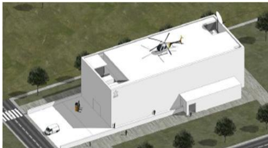
New bunkerized On-site Emergency Control Centre
