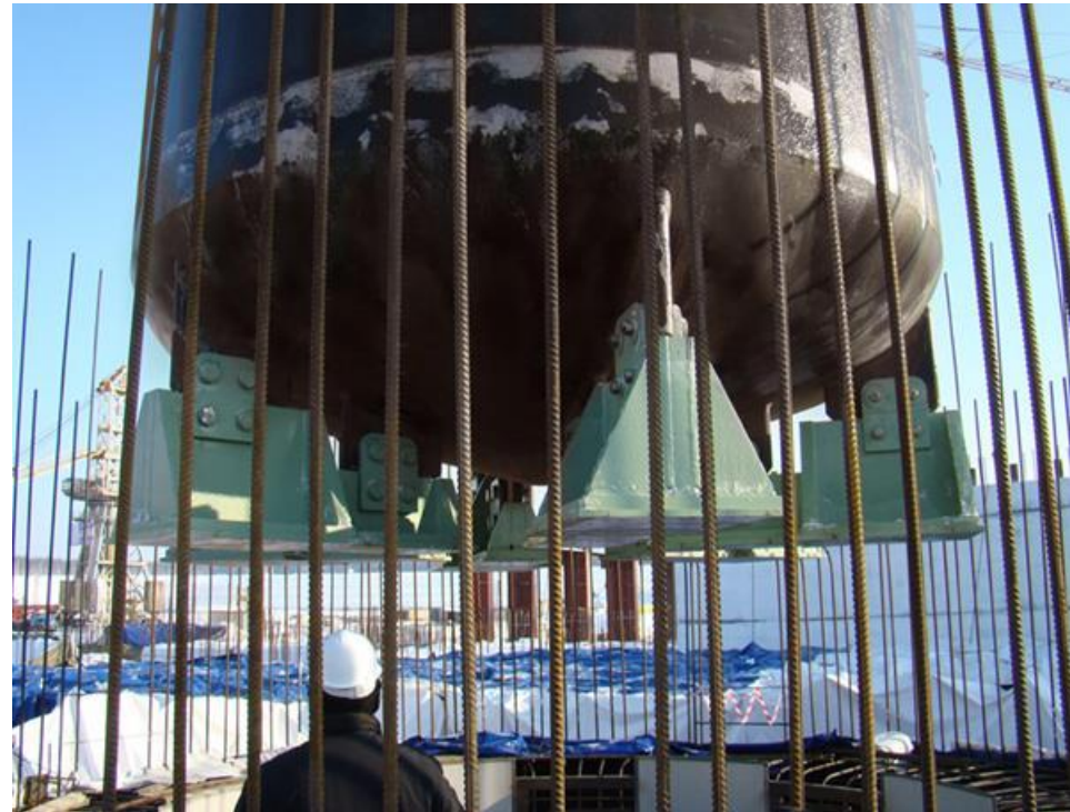
Installation of the shell of the core catcher
