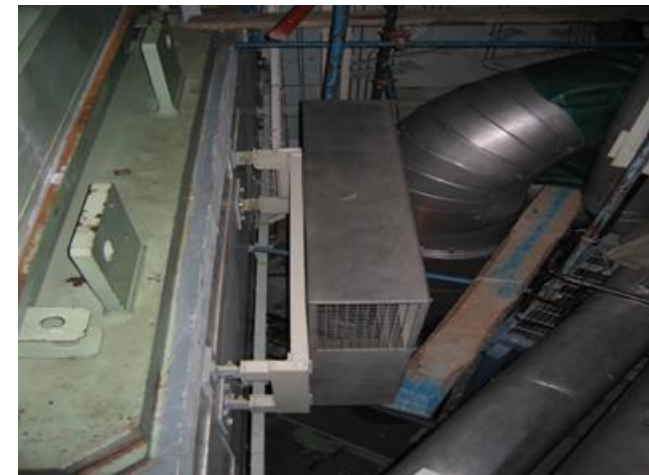
Passive catalytic hydrogen recombiners at operating VVER
