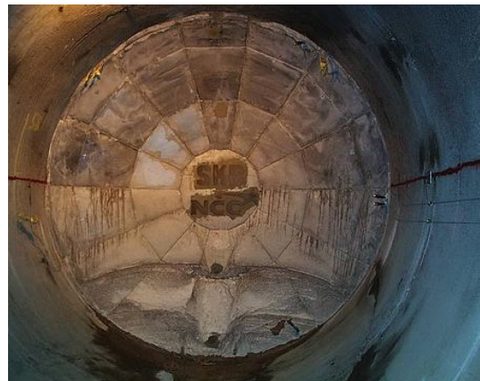
Concrete tunnel plug (Sweden)
