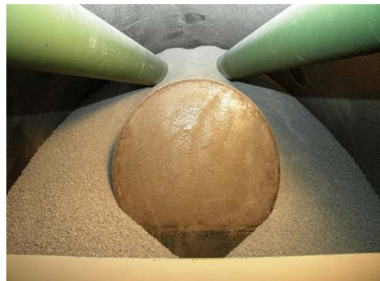
Granular backfill emplacement (Switzerland)
