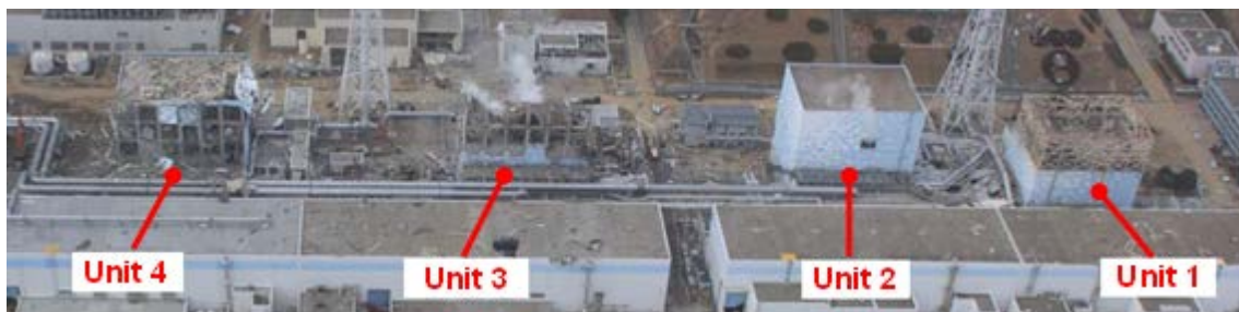
Figure 16: View of the reactor buildings following the explosions [38].
