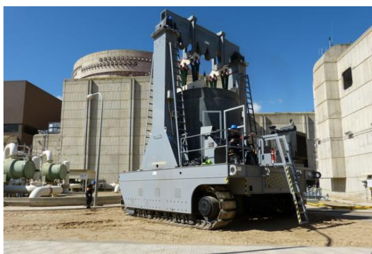
Figure 6. Cask transfer at Ascó NPP site
