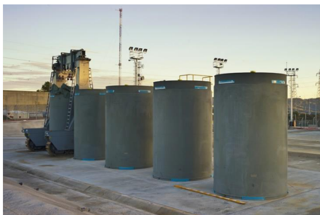
Figure 5. ISFSI at Ascó NPP site
