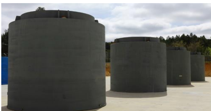
Figure 4. ISFSI at José Cabrera NPP site
