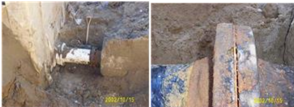
Figure 21: a) Corroded Elbow, b) Leak Area Wall Thickness Measurement, c) Underground Buried Pipe Coupling Connection, d) Anti-Corrosion Tape
