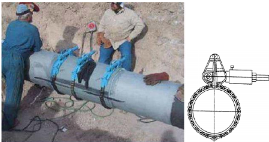
Figure 2: “Type A” Welded Sleeve Repair Techniques
