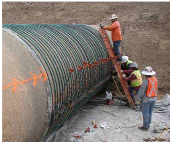
Figure 8: Post-Tensioning Repair
