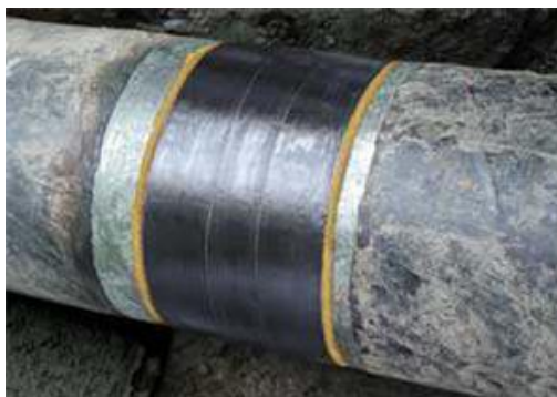
Figure 6: Carbon Fibre Wrap Repair
