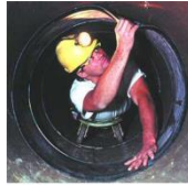
Figure 4: Weko-Seal® Repair
