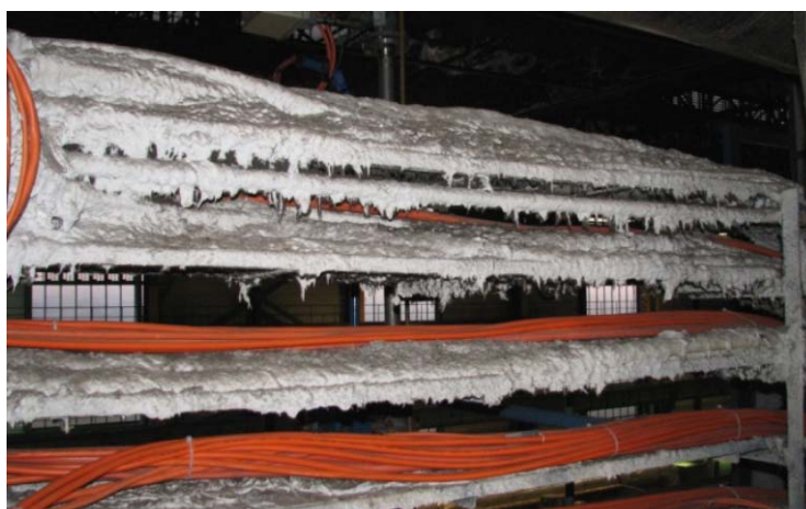
Figure 3.3.7-1: Fire protection layer for cables
