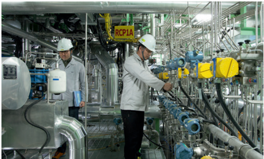
The ATLAS facility. KAERI, Korea
