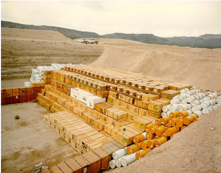
Figure 4.10: Typical low-level radioactive waste emplacement in a trench at the Nevada Test Site (now called the Nevada National Nuclear Site)
