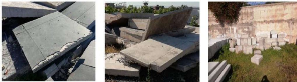
Figure 3.5: Grid of the LNS 20 and 40-degree experimental room (left) and Magnex experimental room (right), involved in the demolishing of the concrete shields. In order to determine the samples for the floor sample, one of every two cubic meters of concrete and for the blocks one cubic metre for every two adjacent blocks have been taken.
